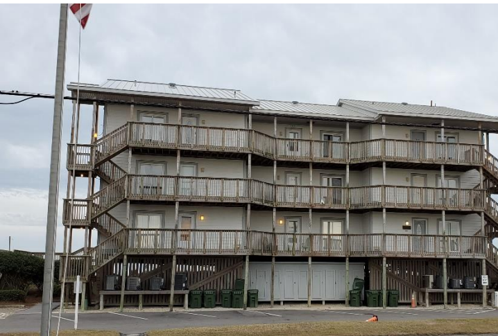
NEW ROOF ON BUILDING A
